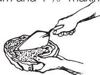
Figure 7 Mortar applied to the entire back of the stone.
